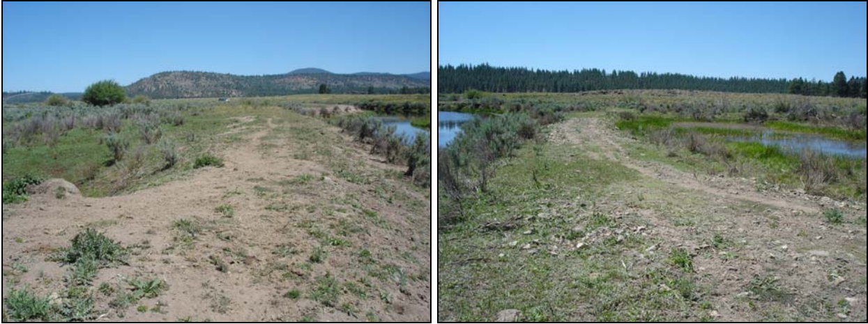
Figure 5-1. Two potential fill removal sites on the Kronenberger reach of the Sycan River. Site 6 (left) is characterized by poor vegetation conditions and floodplain confinement. Site 10 (right) separates the river from an off-channel wetland.
