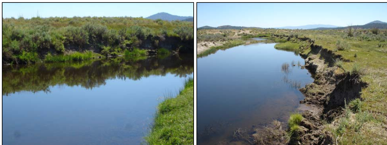
Figure 5-3. Two sites characterized by vertical bank failures related more to fluvial processes than livestock access. Site 4 (left) is a short reach characterized by a vertical-to-overhanging bank. Site 9 is a more extensive reach characterized by an eroding outside bank that is contributing large blocks of soil to the river (right). Sloughed blocks may stabilize at the bank toe and revegetate as seen in the middle ground of the right photo.
