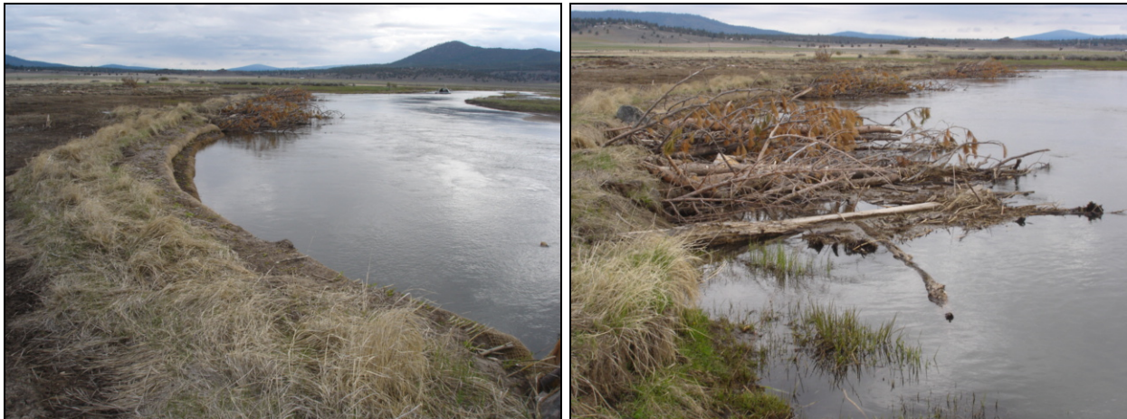
Figure I-6. Example bioengineering (left) and engineered log jams (right) on the Sprague River. Bioengineering and log jams provide bank stability and diverse aquatic habitat. Over time, the willows planted in the soil lift will form a dense willow thicket.
