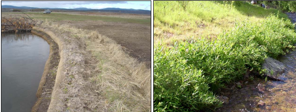
Figure I-8. Examples of soil lifts on the Sprague River (left) and Belmont Creek (right). The Sprague River photo was taken in the spring following installation. The Belmont Creek photo was taken 2 years after installation.
