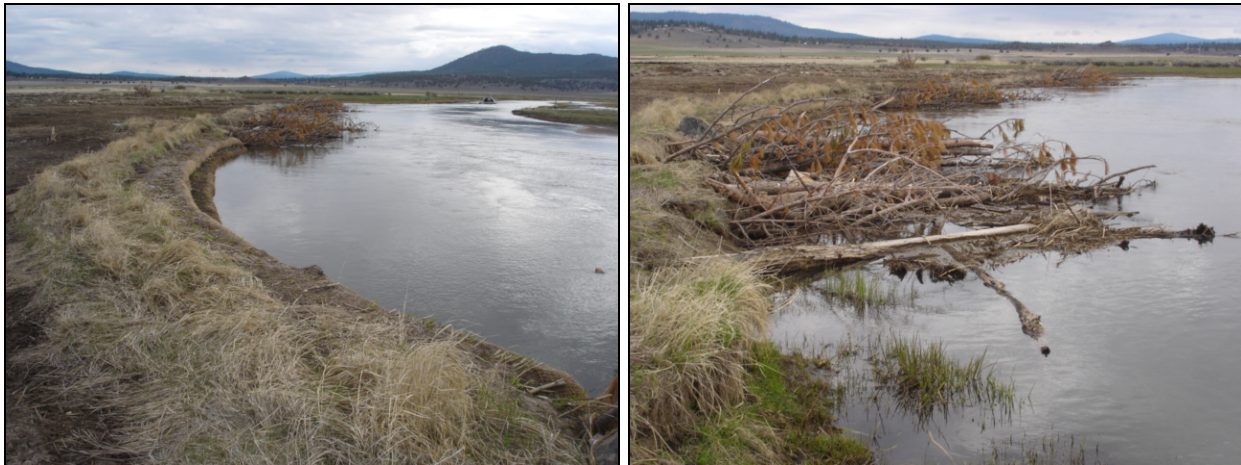
Figure 4-6. Example bioengineering (left) and engineered log jams (right) on the Sprague River. Bioengineering and log jams provide bank stability and diverse aquatic habitat. Over time, the willows planted in the soil lift will form a dense willow thicket.
